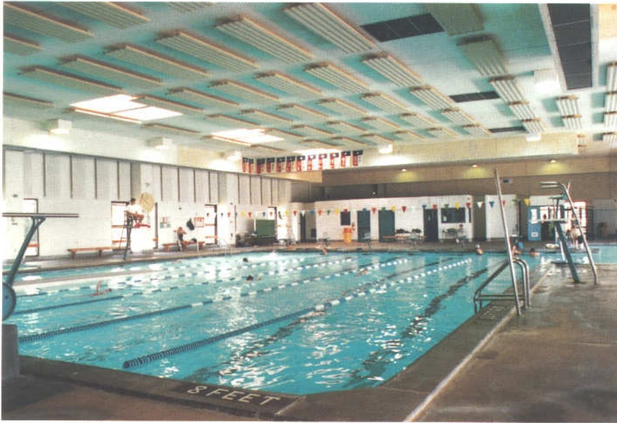
Eckel noise control panels can be used in hostile environments such as swimming pools and outdoor environments, often without disturbing existing utilities.
